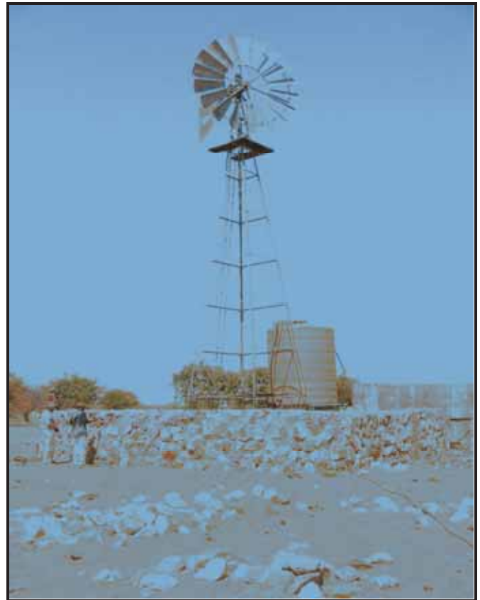
Figure 1. Successful protection wall against elephant at a water point in #Khoadi //hoas Conservancy, Kunene Region, Namibia. Photo: Olga Jones.
